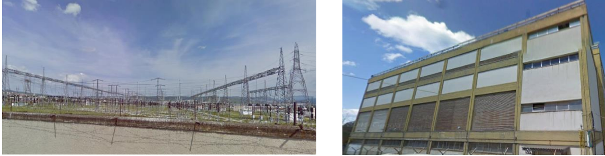
Figure 3: Representative open-type (left) and close-type (right) substations [Google Maps]
