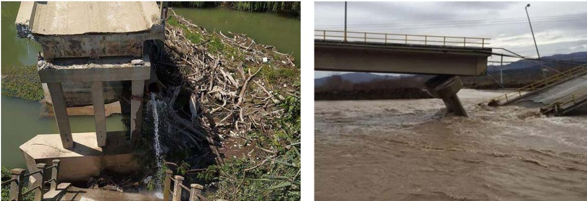
**Figure 1.** (Left): Bridge failure due to flood and accumulated debris (Serres, Greece). (Right): Bridge failure due to flood, causing deck unseating (Kalampaka, Trikala, Greece)
