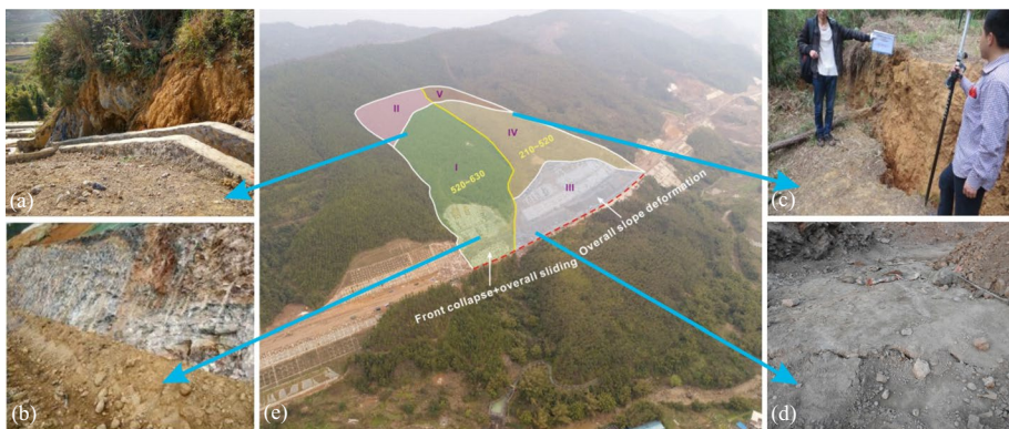
Fig. 2 On-site investigation of the landslide area: a landslide bed, b shear outlet, c steep scarp and d uplift of road surface
