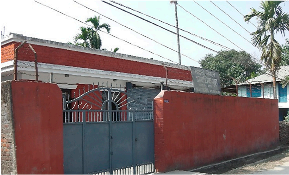
Figure 2. One shelter home along Indo-Nepal borders.
