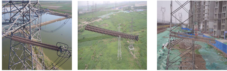
Figure 6. Sample images of CPLID dataset, containing normal insulators images ( left side ) and synthesized images of insulators with missing cups with diverse backgrounds ( center, right side ).
