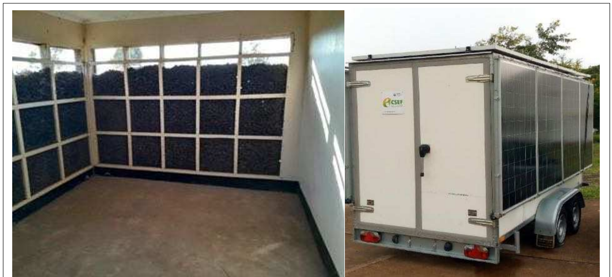
Figure 1: A charcoal cooling room (left) and a walk-in, mobile, solar-powered cold storage unit (right) for storing fresh vegetables
