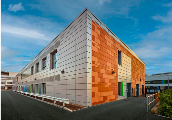
(b) The completed ward
