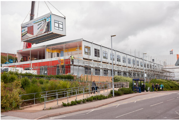
(a) Modular units in construction
