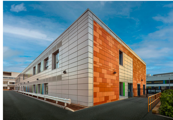
(b) The completed ward
