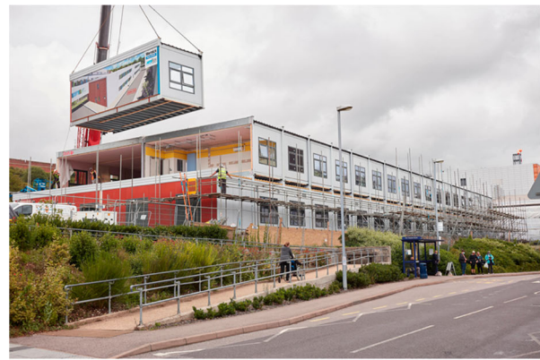
(a) Modular units in construction
