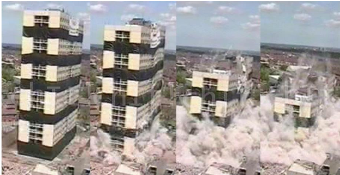
Figure 1. Implosion of Kenley Tower.
