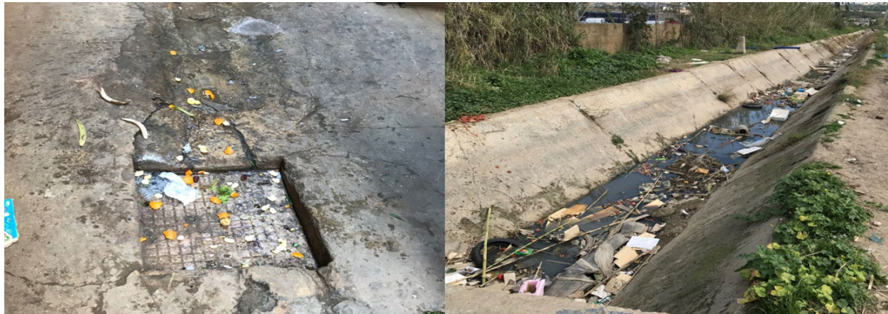
Figure 3-4. PCS Hygiene Observations. Waste scattered inside the PCS building between household units (left). Contamination of the Litany River branch near the PCS (right).
