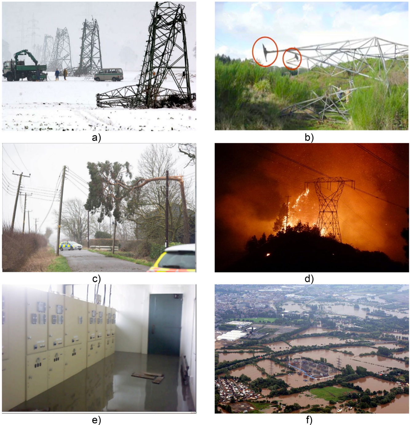
FIGURE 3 | Failure modes of power grid sub-systems against natural hazards: (a) tower collapse due to compounding ice and wind (Spiegel 2005); (b) footing failure of the tower due to wind (Eidinger and Kempner 2012); (c) damage to distribution network due to fallen trees (BBC 2020); (d) damage to transmission network due to forest fire (RTO 2021); (e and f) equipment malfunction due to indoor and outdoor substation inundation (Eidinger 2011) and (National Grid 2016).
