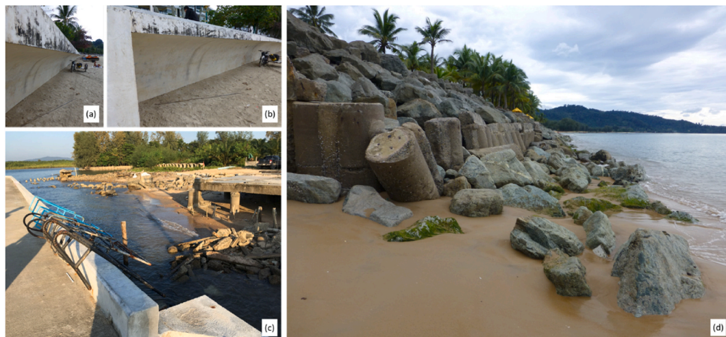
Fig. 16. (a) and (b) Recurved concrete seawall in front of the Seagull at Southbeach apartments in Patong Beach; (c) Baan Nan Khem pier; (d) severe erosion at the toe of concrete revetment (Lat 8° 40' 3.13" Long 98° 14' 34.87").
