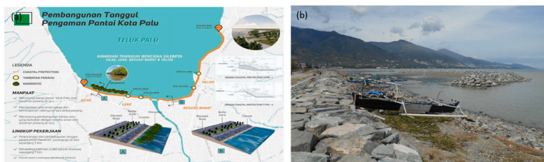
Fig. 15. Palu City coastal defences: (a) Infographic on the Palu Coastal Protection project; the location of the four boat mooring facilities is shown in yellow circles [84]; (b) new revetment and boat mooring facility in Lere in December 2022.
