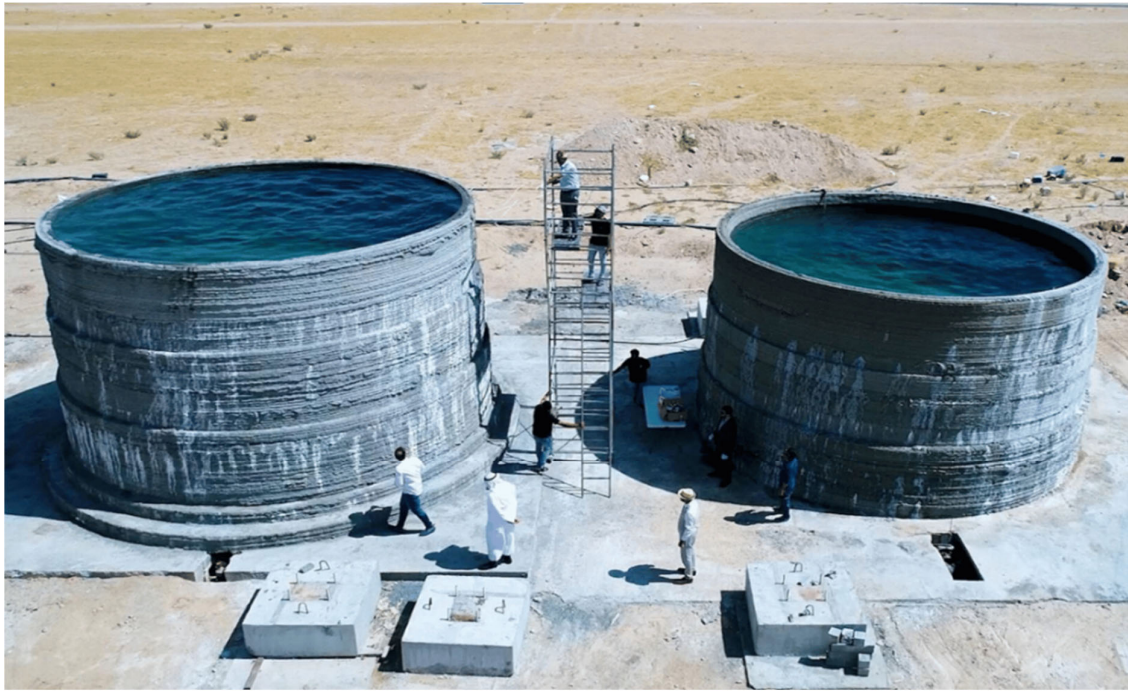
Figure 5. The first on-site 3D printed water tanks in Kuwait by Abyan Building Construction Company.
