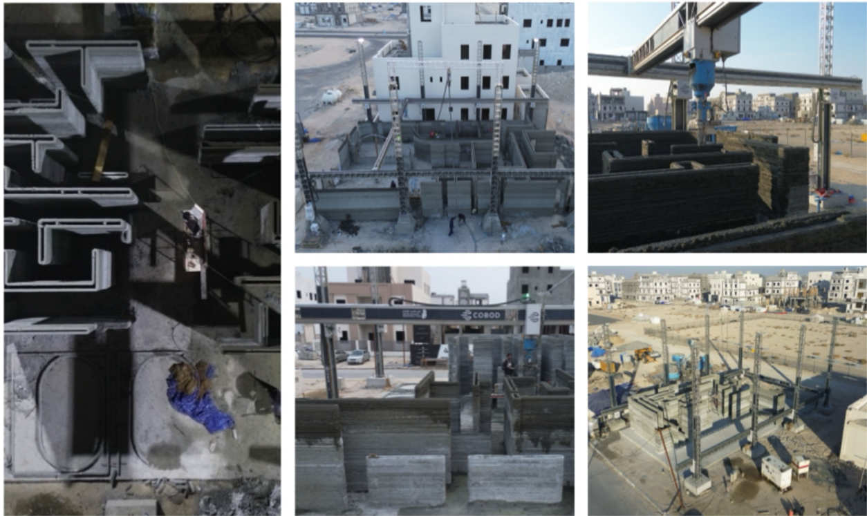
Figure 4. The first on-site 3D-printed house in Kuwait by Abyan Building Construction Company.
