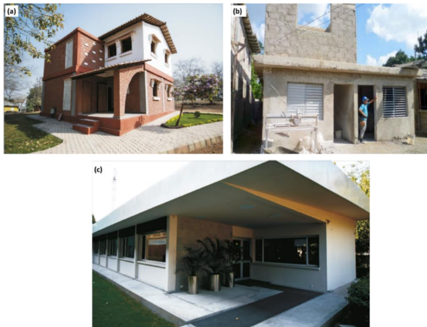
Figure 2.11. Constructed LC3 buildings (a) Model house in Jhansi, India, (b) Model house in Santa Clara and (c) building at the Swiss embassy in Delhi, India [155]
