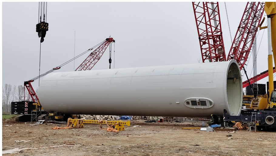
Figure 2.11: Tower, supports the entire turbine structure and elevates the rotor and nacelle to an optimal height to capture more wind energy.
