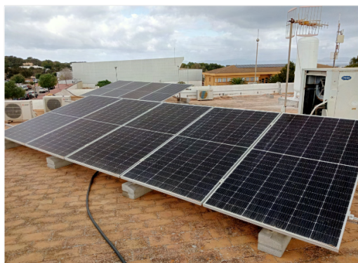
(a) New 15kW rooftop solar installation on the Community Centre
