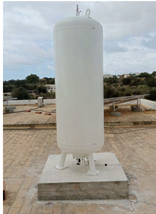
(b) Installation of the 1,000 litre hydrogen pressure vessel.
