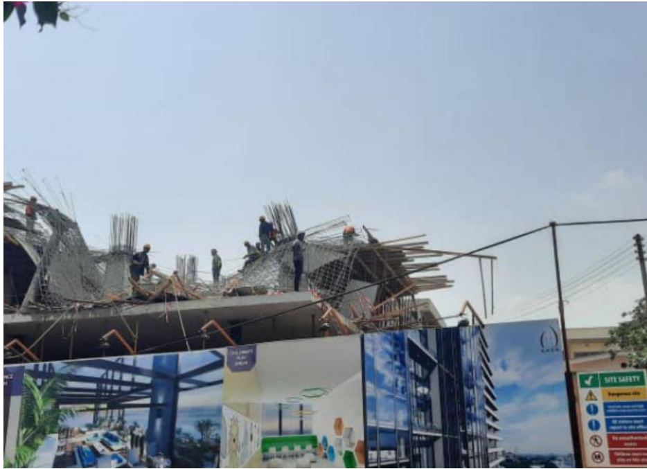
Figure 1.1 A section of a 22-storey building under construction at the Airport Residential Area, near Association International School (Menz, 2021)
