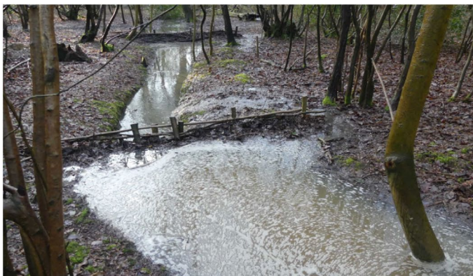
FIGURE 2 | Group of leaky woody dams in Ruislip Woods (left). Standard basic “design” of a LWD (right).
