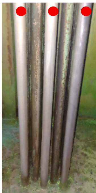
Fig. 20. Monel 400 pipes after cleaning (only pipes marked with red dots were cleaned) in condensation unit section no. 1. (For interpretation of the references to colour in this figure legend, the reader is referred to the web version of this article.)
