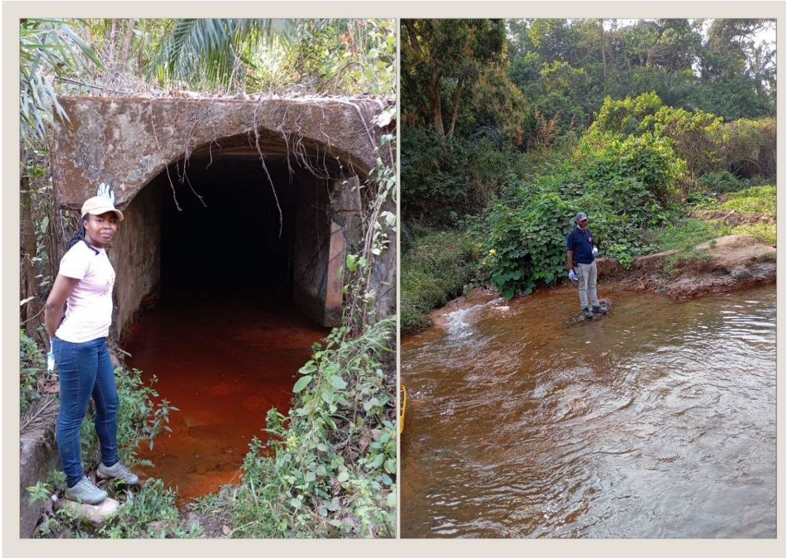
Figure 2.3: Point source pollution from the Onyeama abandoned mine adit discharging into the Ekulu River tributary
