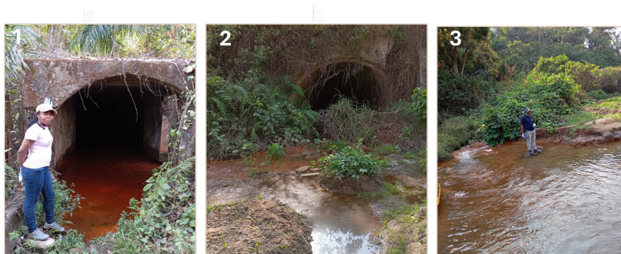
Figure 6.6: Mine water discharge points at the abandoned Onyeama coal mine. (1) Tunnel 1 (Adit 1), (2) Tunnel 2 (Adit 2), and (3) surface flow between the two tunnels. The orange colouration indicates the influence of acid mine drainage and iron oxide precipitation.
