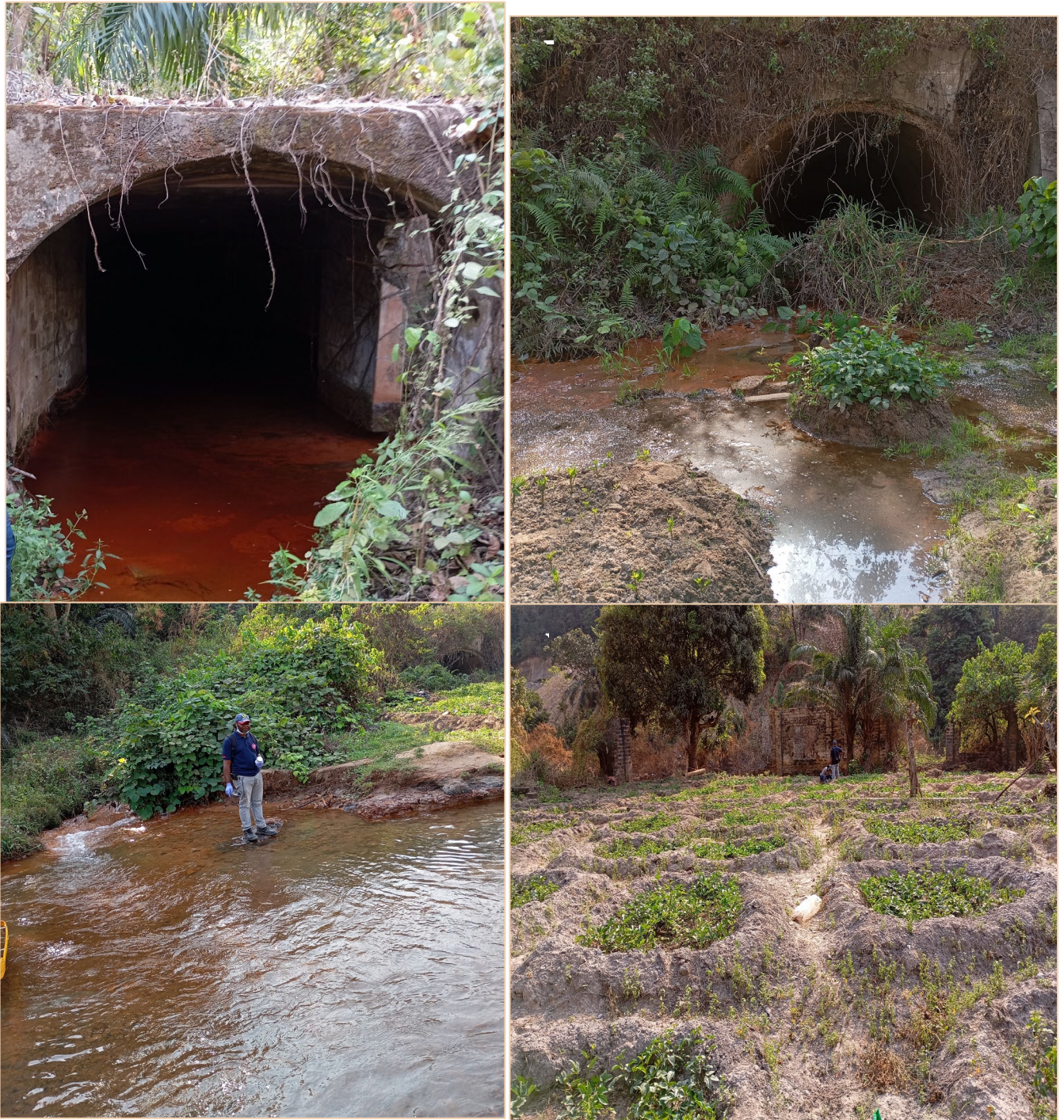
Figure 6.4: Onyeama Abandoned Underground Coal Mine. (a) Mine Adit on the left wing with acid mine drainage flowing into a stream; (b) second mine Adit on the right discharging into a stream; (c) receiving stream from both mine Adits; (d) mine area currently used for agriculture, with vegetables planted within the ridges.
