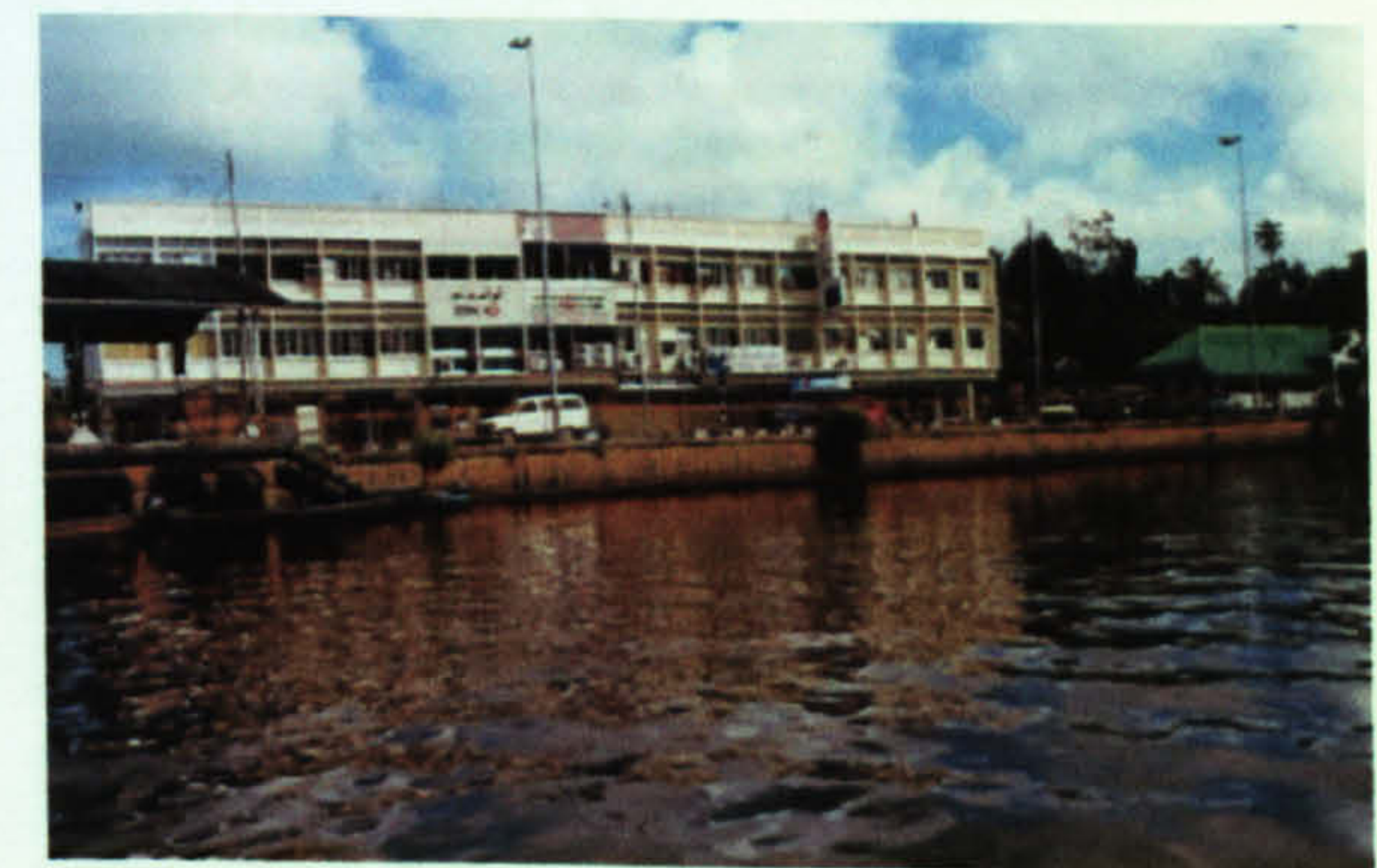
Plate 3.7.6 Tutong River - A town jetty, probably moderate source of pollution.
