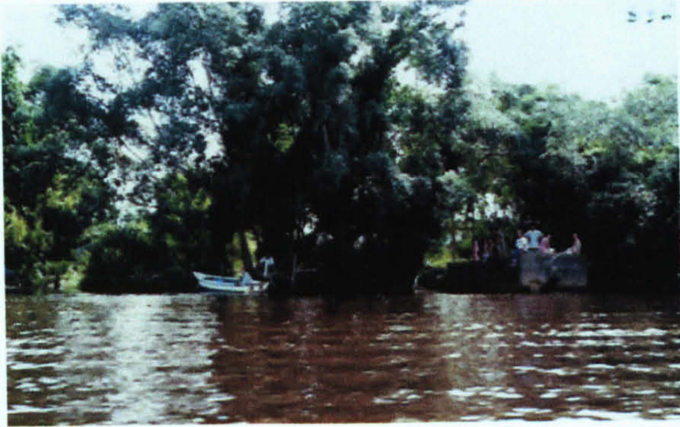
Plate 3.6.1 Belait River - Old sewage treatment area
