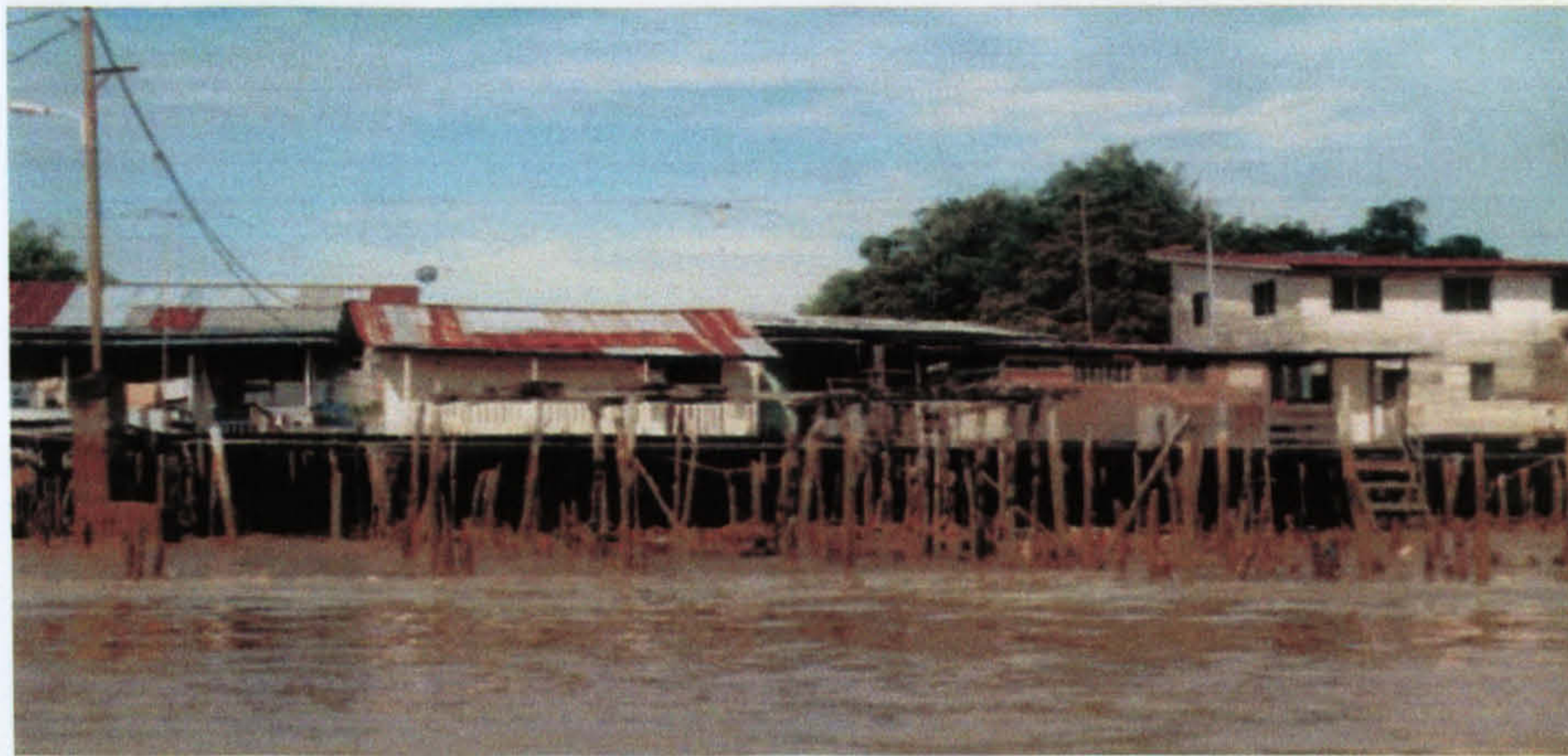
Plate 2.6.2 The roof tops from the wooden houses in water village which is made from zinc and the stilt made from concrete or iron bars.
