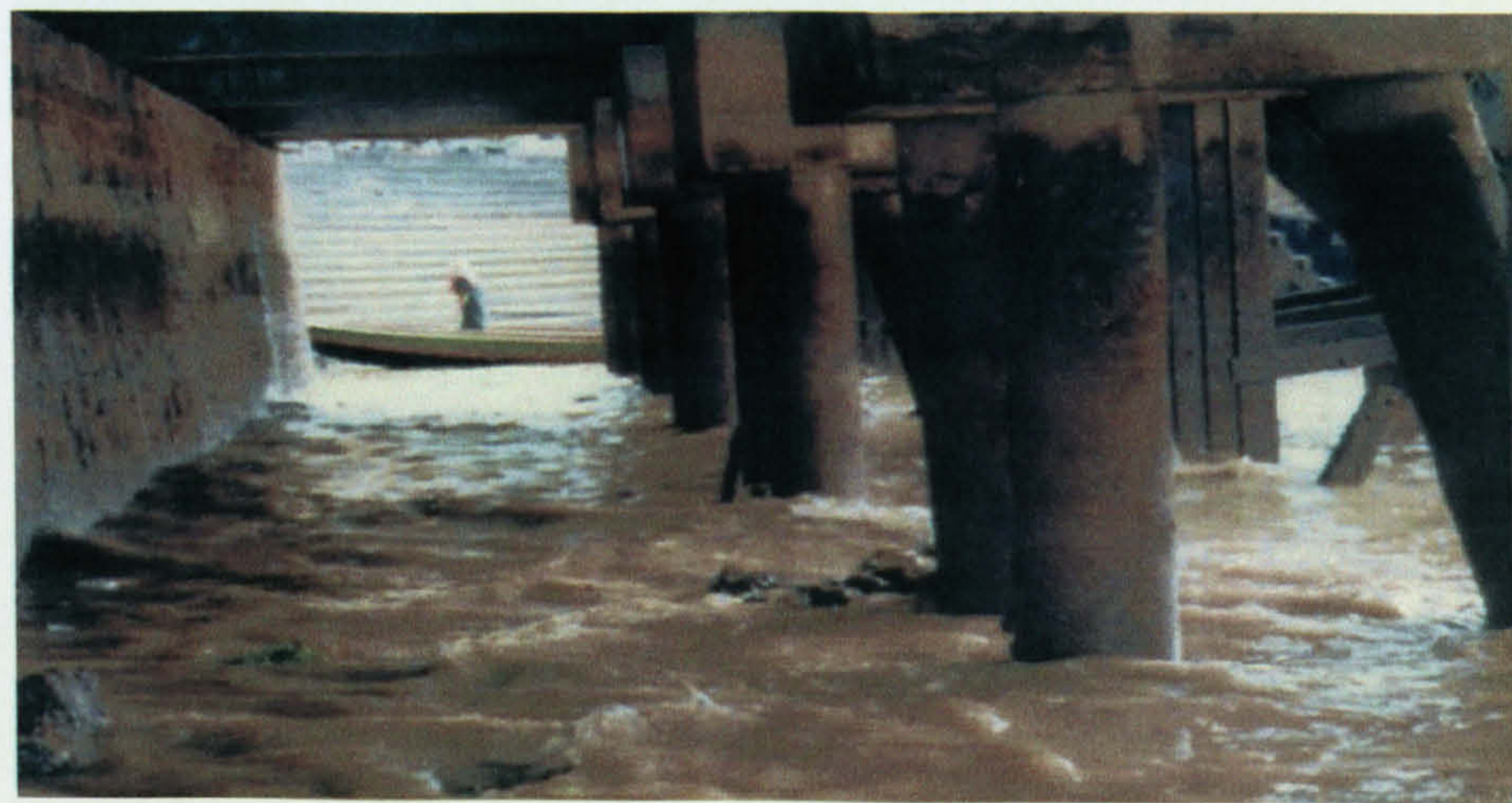
Plate 2.6.3 A closer view of stilt concrete.
