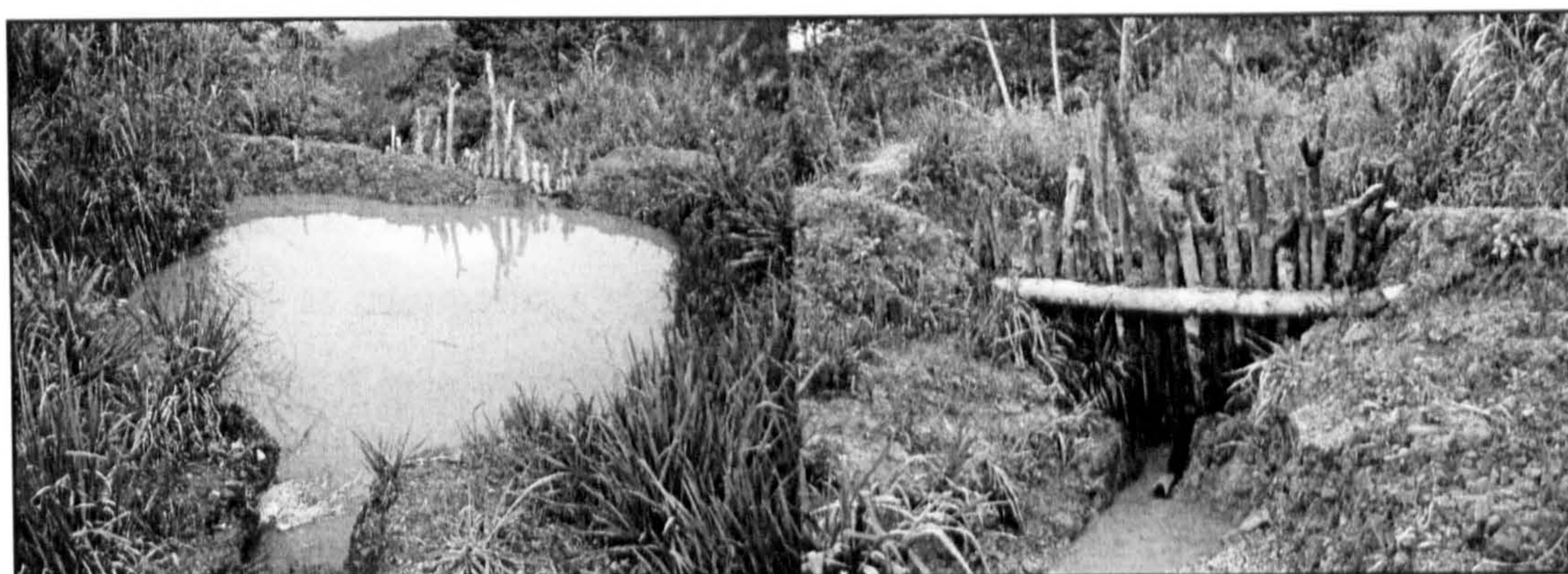
Figure 15. A mining pond (left) with a close-up of its “vertical stakes”-type dam (right).
