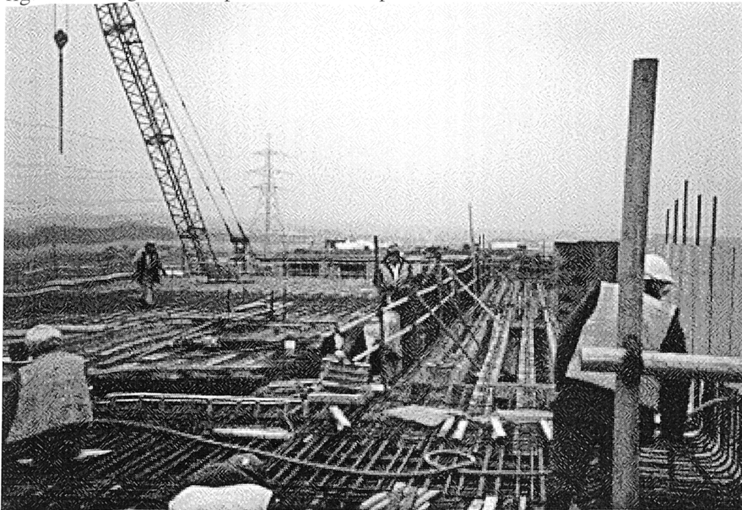
fig. A.1. Bridge surface prior to concrete pour.
