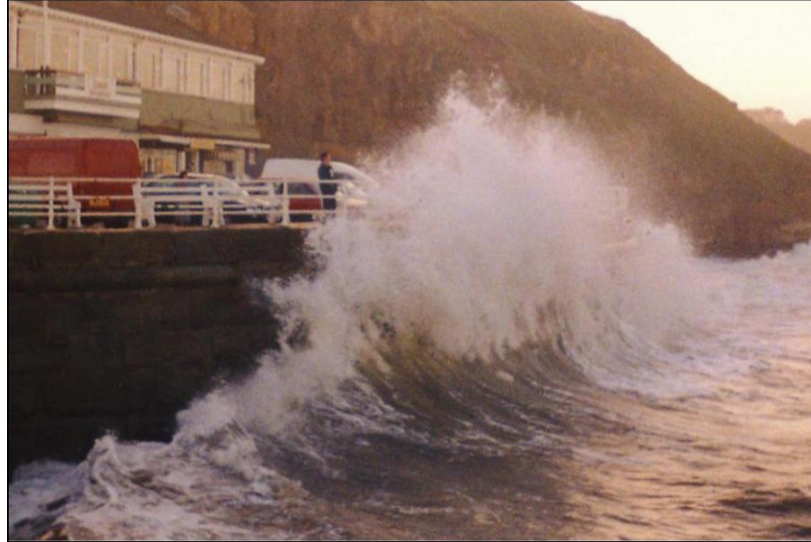
Figure 2.7.1: Overtopping at Whitby, UK, image taken from
