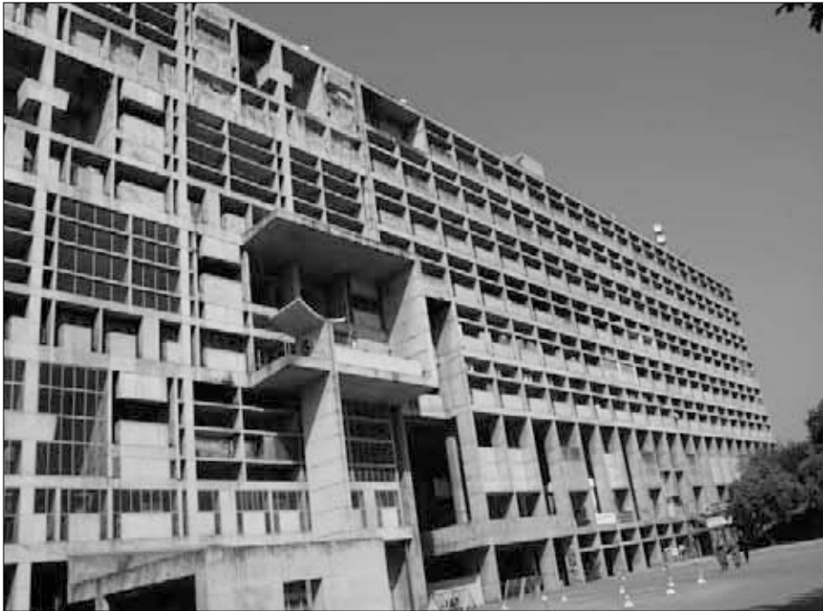
Figure 9: The Brise Soleil Façade of the Secretariat, Chandigarh
