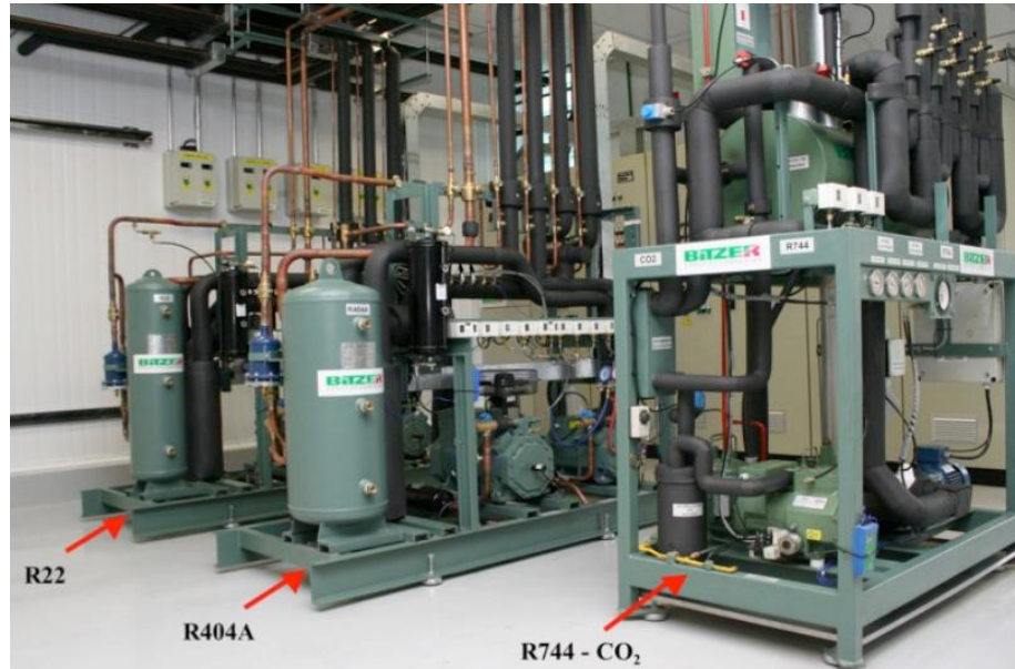
Figure 2.22 Image of CO 2 /R404A Cascade, R22 and R404 refrigeration systems trailed by Bitzer for supermarket refrigeration (Silva et al. , 2010)
