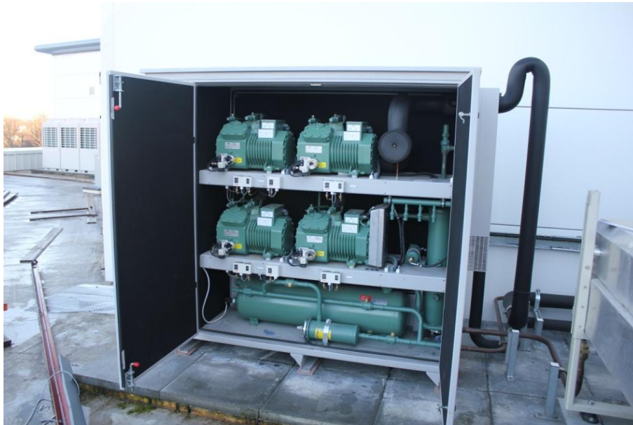
Figure 7.5 MT refrigeration multi-compressor pack system
