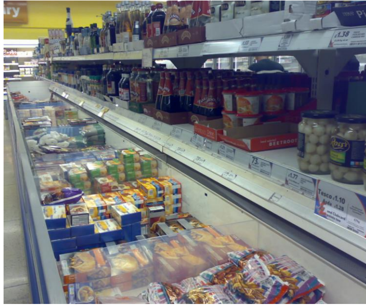
Figure 2.3 Horizontal (well) type cabinet
