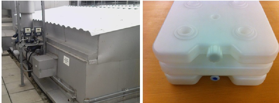
Figure 3.1 PCM tank. Roof-mounted PCM tank (left) and stacks of FlatICE containers as they would be found inside (right).
