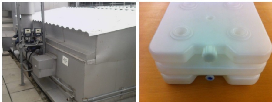
Figure ES.2 Active PCM storage. One of the roof-mounted PCM tanks (left) and a stack of PCM containers (right).
