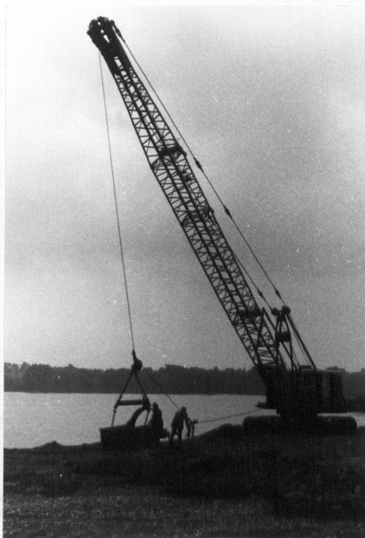
Fig. 13 Crane and bucket dragline.
