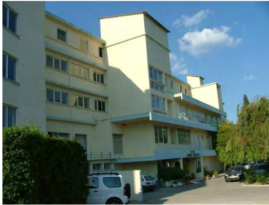
Figure 1 Southeast orientation (circulation areas to the rooms)
