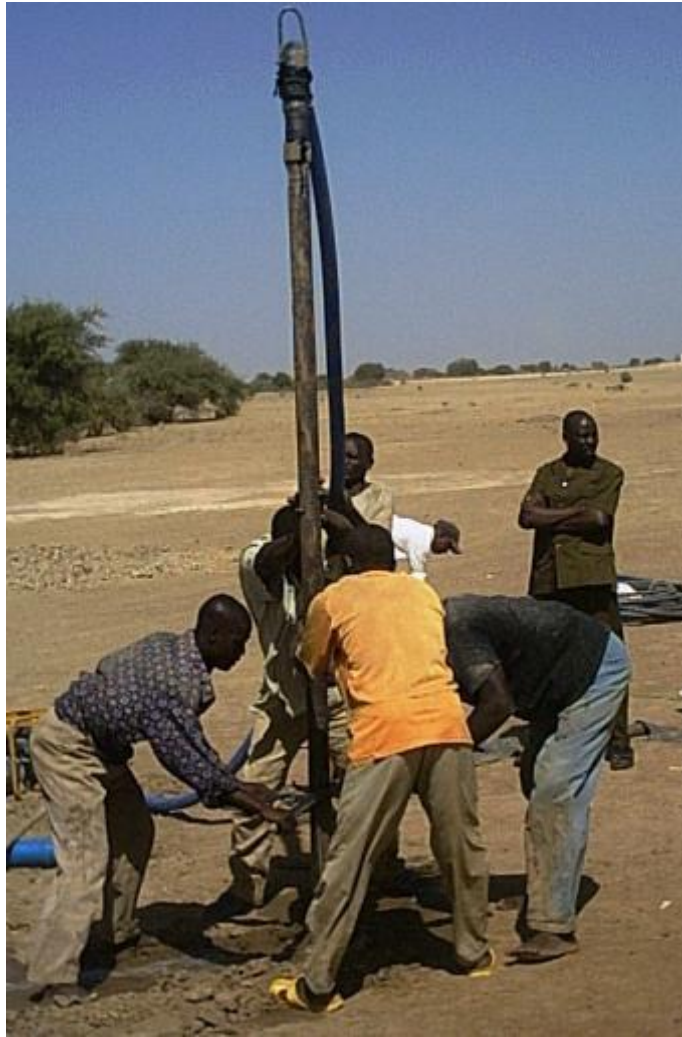
Figure 2.16: Jetting hand-drilling technique (RWSN, 2013).
