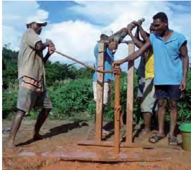
Figure 2.14: Hand sludging drilling technique (Labas et al., 2010).
