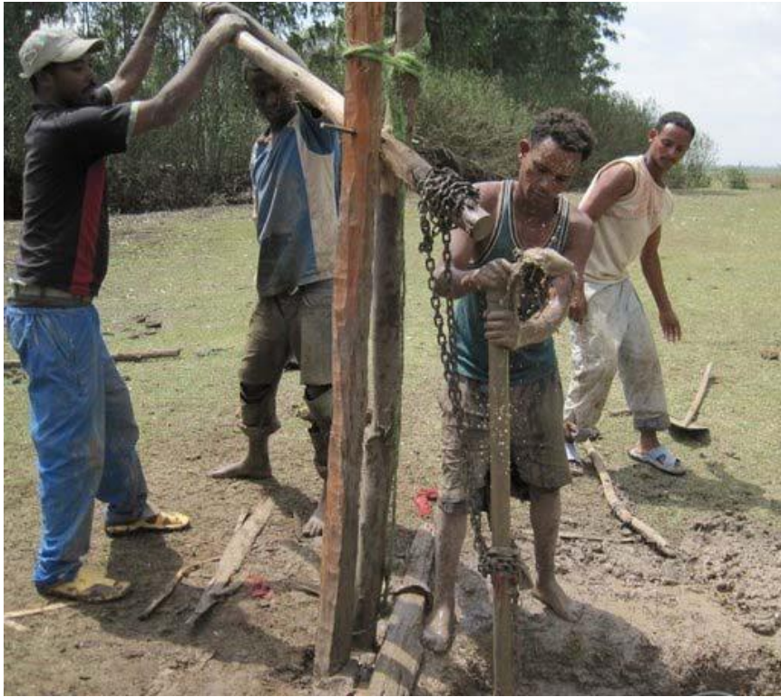
Figure 2.15: Rota sludge hand-drilling (Weight et al., 2012).
