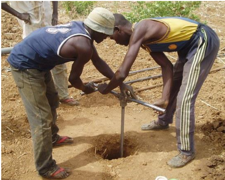
Figure 2.12: Auger hand-drilling technique (RWSN, 2009).
