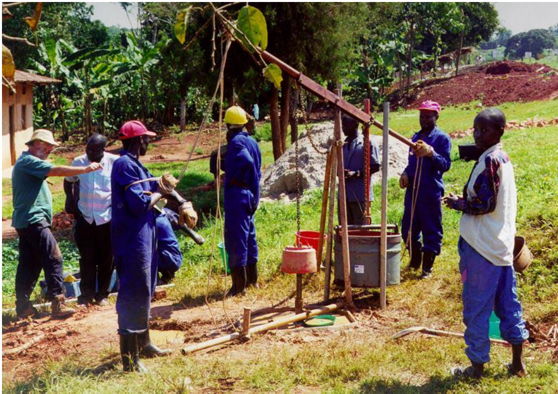
Figure 2.20: Pounder rig hand-drilling (Ball and Danert, 1999).
